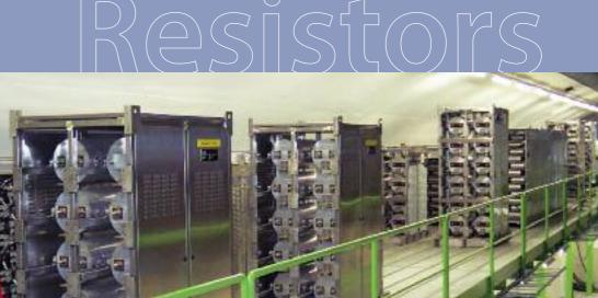
Braking Resistors for large motors are customised to best comply with any requirement: we have developed special Braking Resistors for important research institutes (among them Max Planck Institute) and for energies in excess of 3400MJ.
