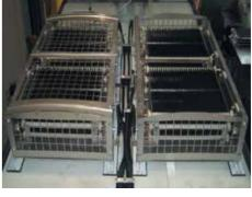
Stainless steel is also used for bolts, nuts and washers. The resistors are designed to avoid disturbing noises caused by pulsating current.
